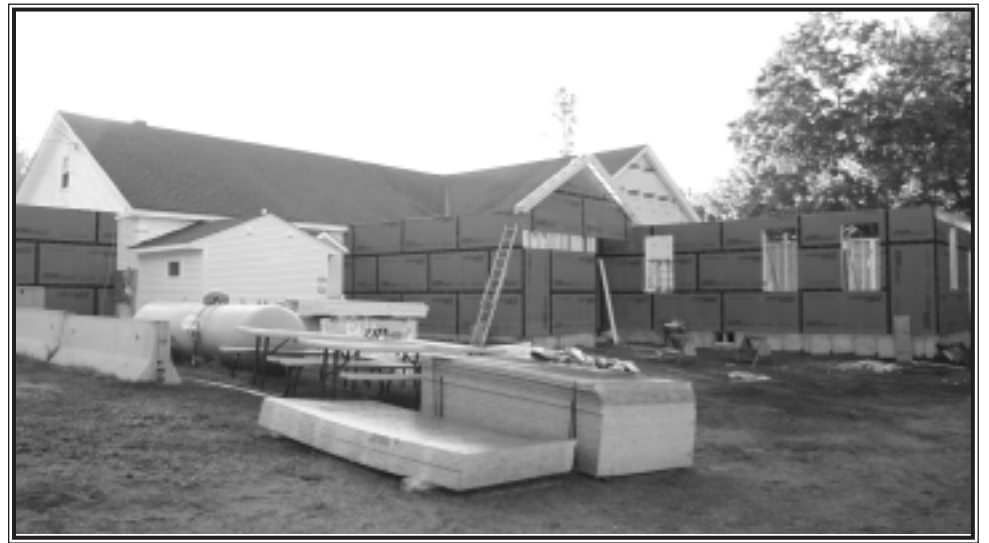
Construction is well under way at the Londonderry Senior Center with the foundations on the additions poured and framing begun. There will be 1,900 square feet added to the existing building. Photo by Chris Paul
